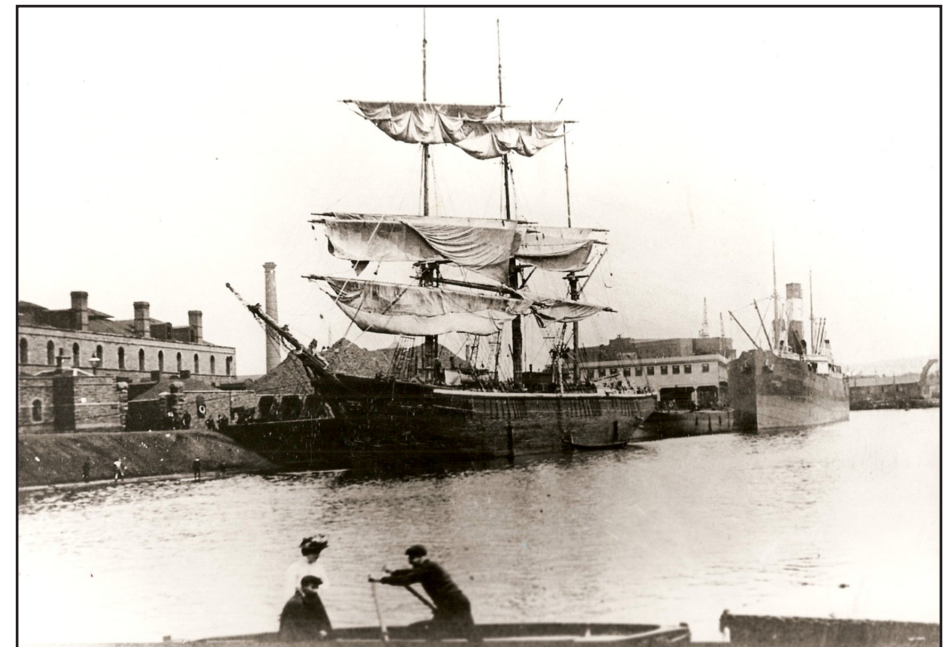
The Mardyke ferry in front of the gasworks. The ferry operated from the middle of the 19th century until 1962, taking shipyard workers to Charles Hills and dockers to the timber yards.
