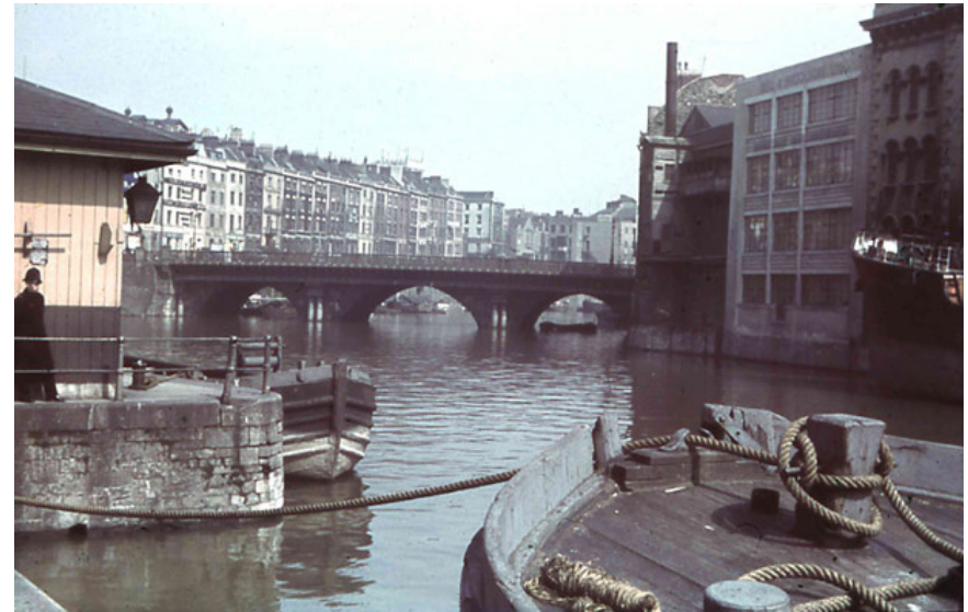
right: The 'new' Bristol Bridge built in 1761 with the metal walkways added by the Victorians to widen it. It was a very busy bridge, for many years the only crossing in the city. This picture was taken in the 1930's, certainly before the war when the buildings beyond the bridge were destroyed in the Bristol Blitz.
